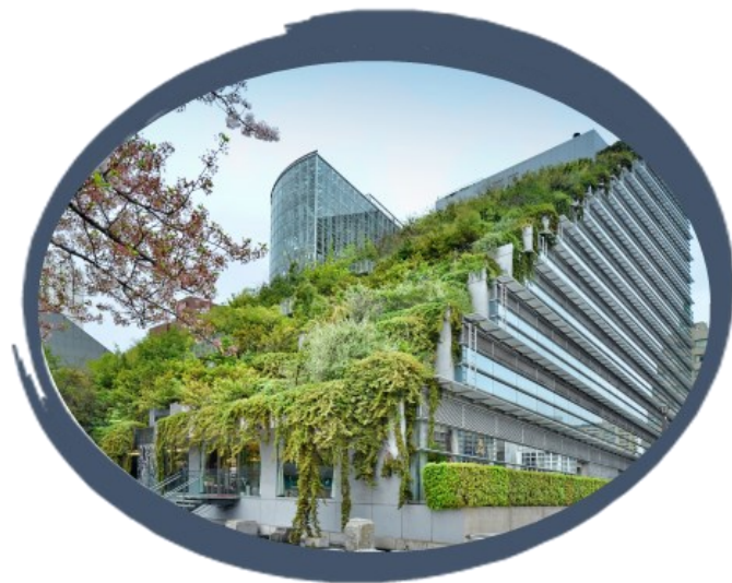
Figure 5: Example of a green roof; Fukuoka, Japan.
