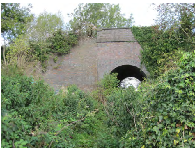
Underpass providing pedestrian route between site and Caldecotte
