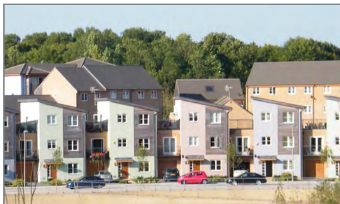
The use of render and light tones helps establish an identity for Ashland
