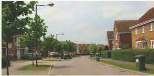
Green "feel" provided by street trees, verges and planting. Importance of street emphasised by street trees and width.
