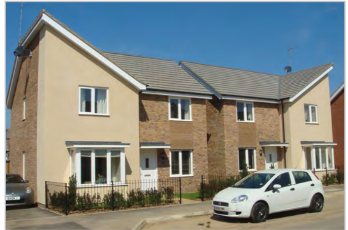
These two buildings have good symmetry and act as 'one'
