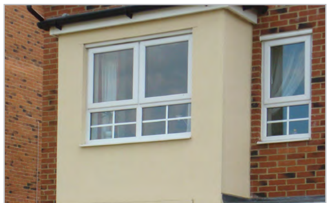
Over fussy glazing bars clutter the elevation
