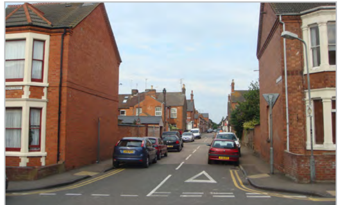
Numerous thin blocks can create inactive frontages along side streets and should be avoided
