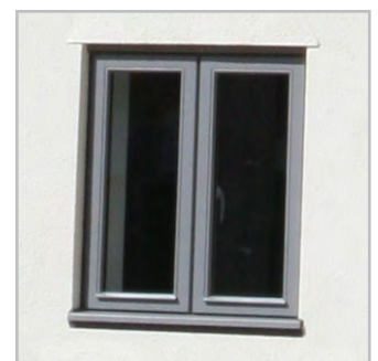
Simple window detailing
