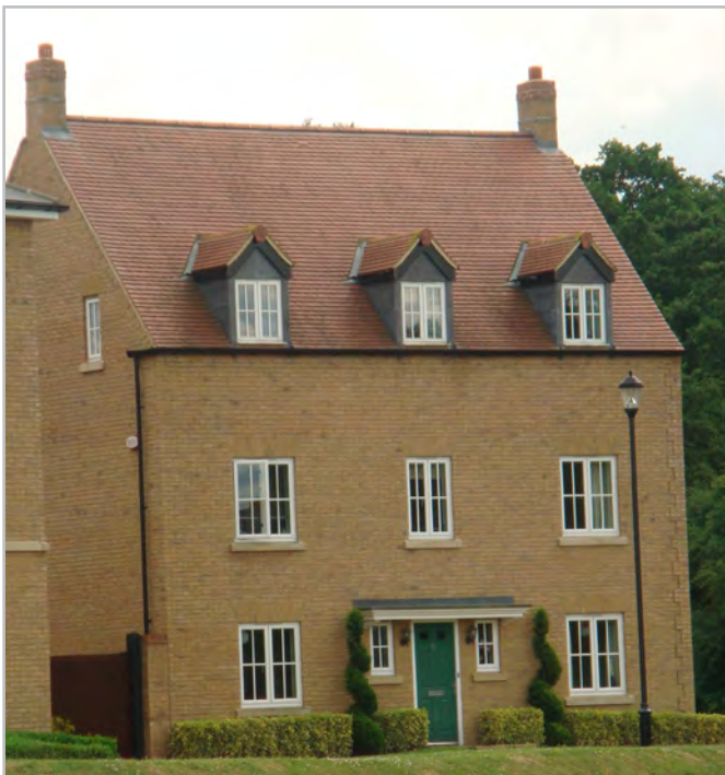
Poorly proportioned building - there is too much of a gap between first floor and dormer windows
