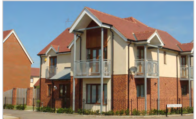
External framed balconies over clutter the elevation
