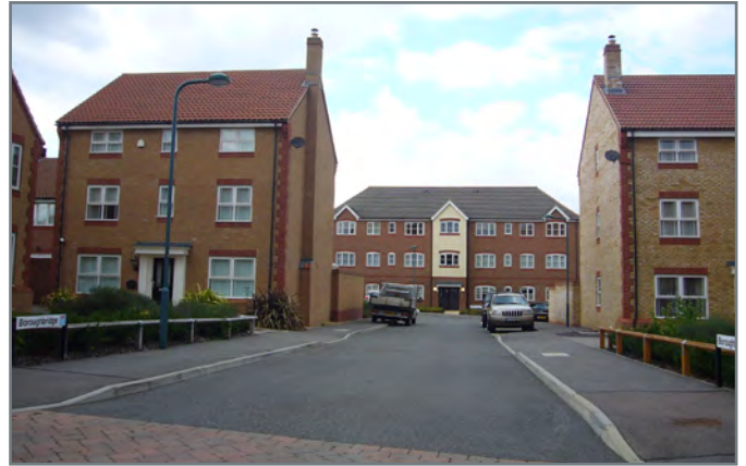
Grange Farm - detailed elevation design has not added to the character of the development
