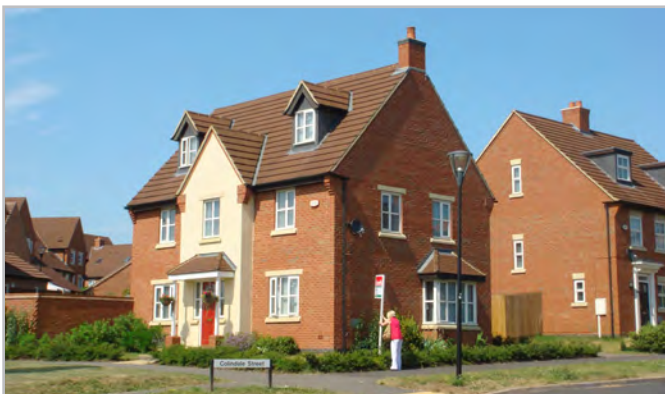
Building turns the corner with active frontage to both streets
