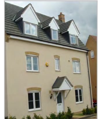
Dormers over-dominate this building.
