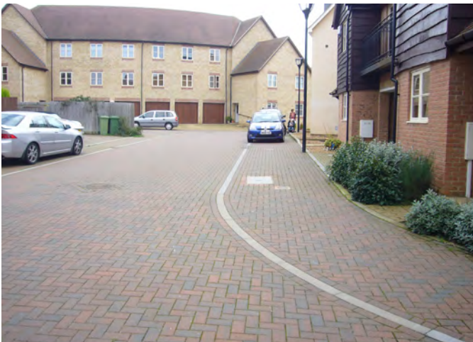
Drainage channels leading to confusion as to whether parts of the level surface are for parked cars or footpaths
