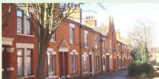
Street with strong sense of enclosure
