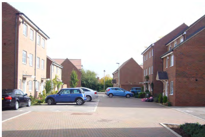
Right-angled parking can serve as a traffic-calming feature
