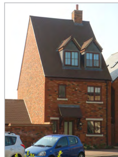
The roof over dominates this house. The location of the dormers furthermore make for poor proportions
