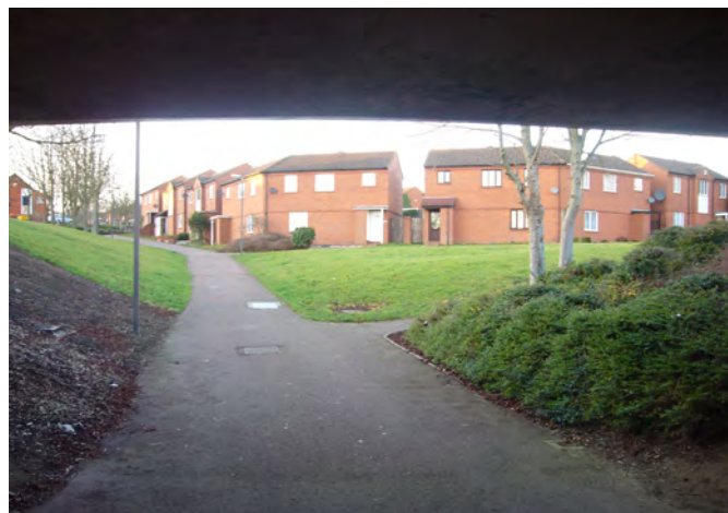
Good surveillance of underpass from neighbouring housing
