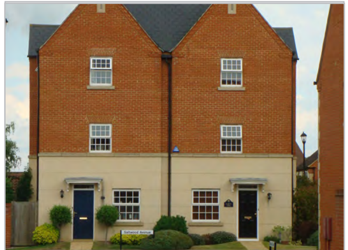
Poor proportion of glazing relative to wall
