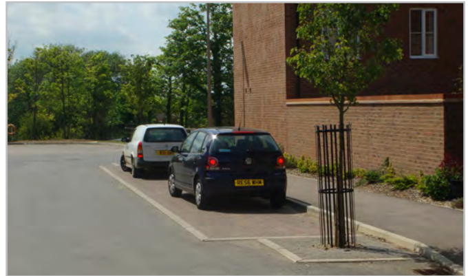
Parallel parking within the carriageway -Woburn Sands
