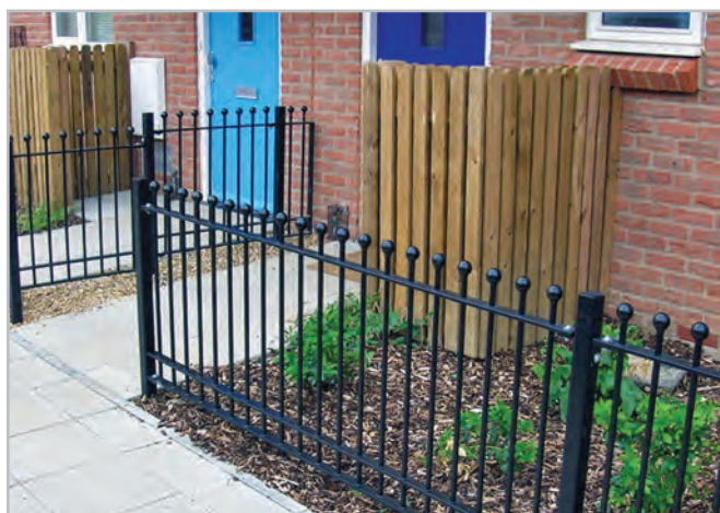
Railings are appropriate boundary treatment in more urban areas
